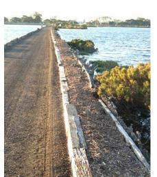
causeway with topping, grading a slope and rolling, organised and assisted by John Gleeson. The concept of making a distinct sloping level to the west is to strengthen and drain the eastern edge against tidal flows in winter.
